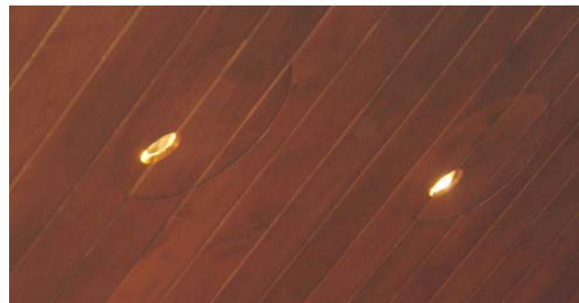
Overlap cover plate in wood ceilings can be recessed as shown or faux painted with wood grain pattern.
