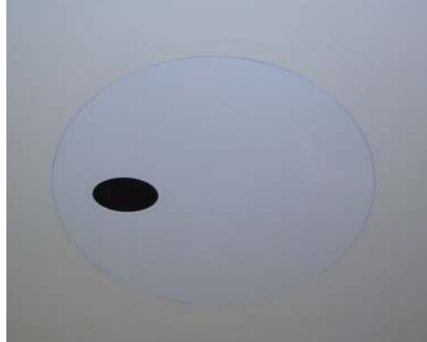
Mud Ring installed in sheetrock ceiling.
